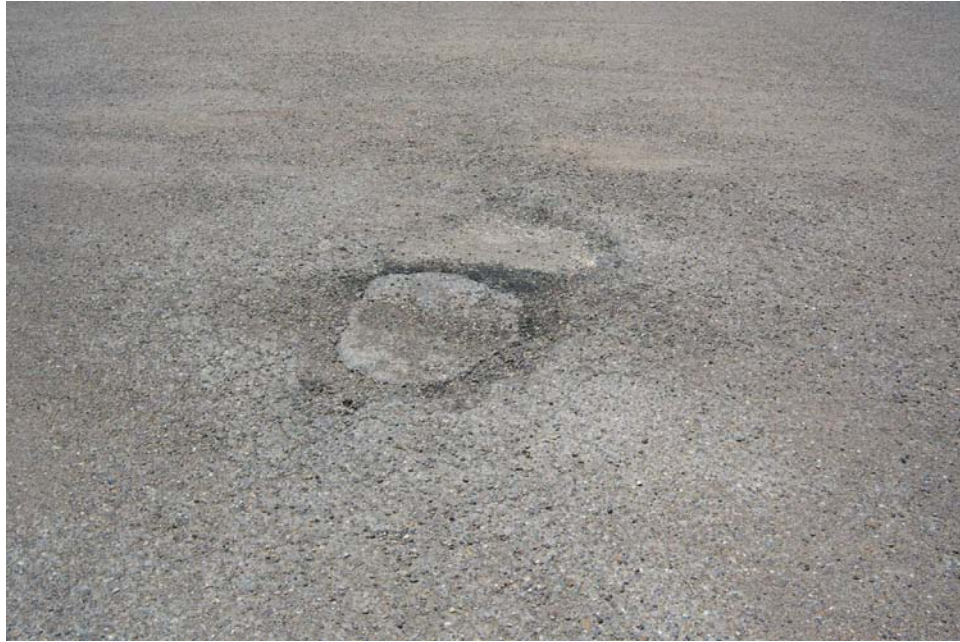
Figure 7 – Parking Lot (Localized Failure)
